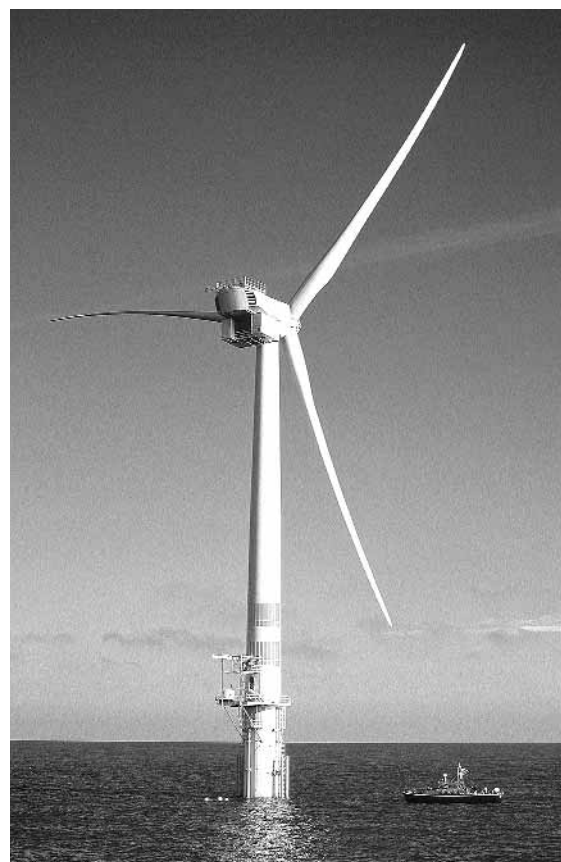
Arklow Bank Offshore Wind Power Facility, Ireland
